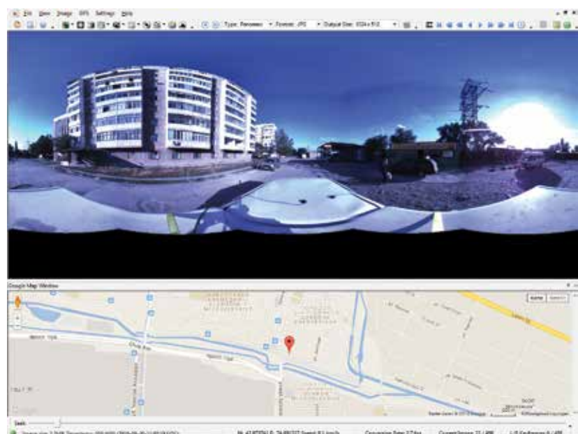
Figure 1. Snapshot of the omnidirectional camera and the buildings captured in the footage as part of the Earthquake Central Asia project.
