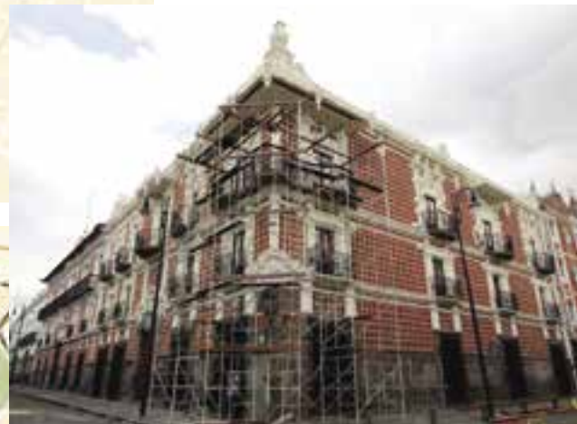
Figure 2. Post-earthquake stabilization of Casa de Alfeñique in Puebla.
