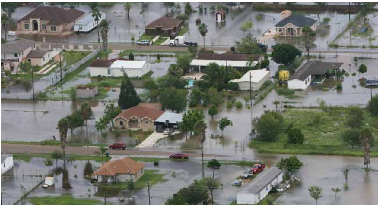
Flooding in Raymondville, another area of Texas prone to floods, during Hurricane Dolly (July 2008). The FEMA floodplain demarcates where development should occur, how high to build structures, and whether to buy flood insurance.
