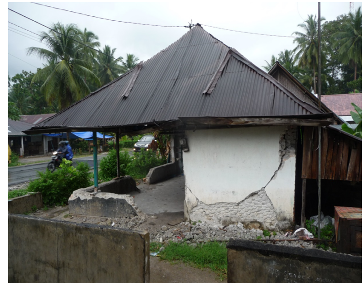
An example of a river rock unreinforced masonry building in Pariaman, Indonesia
