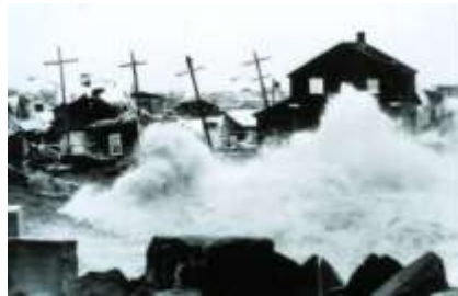
Flood from Storm Surge
