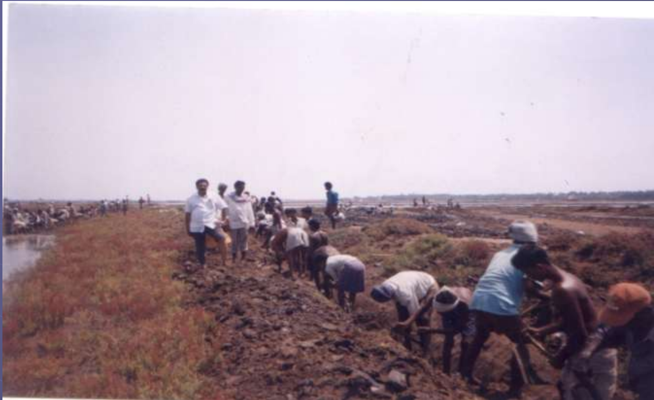
Community at work for Mangrove Regeneration work (channel development).
