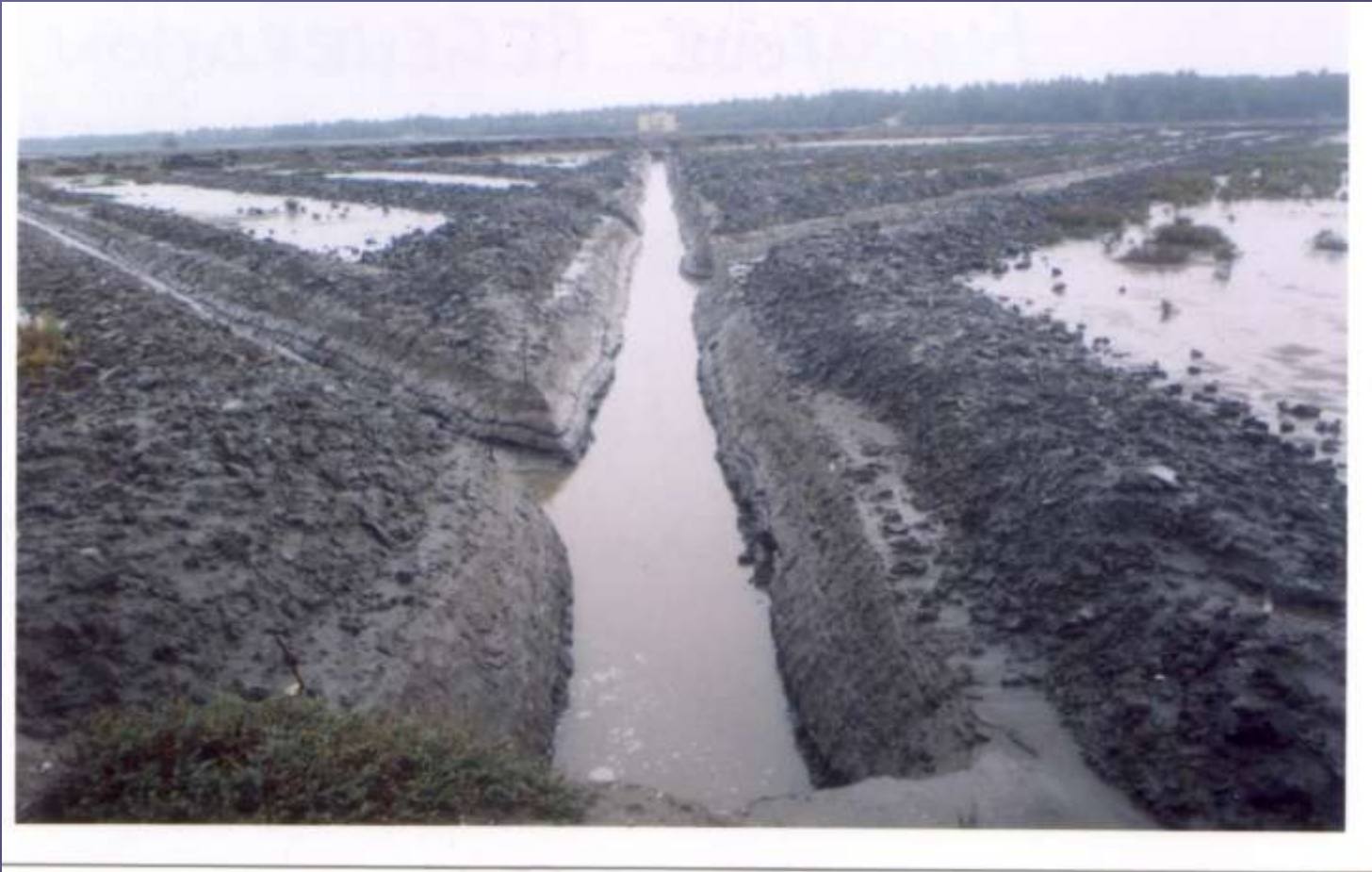
Channeling work for Mangrove Regeneration
