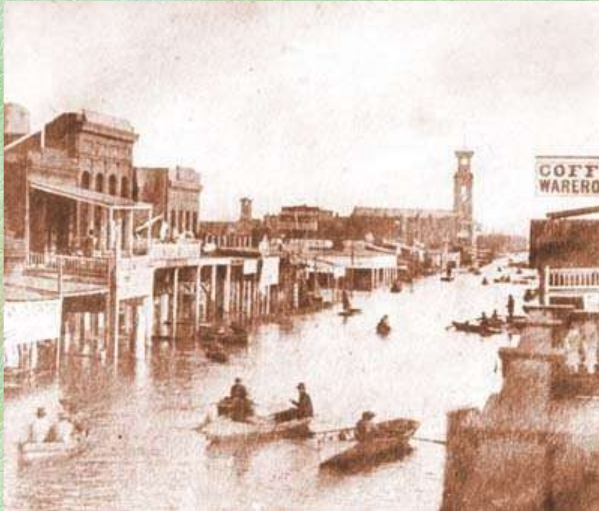
Flooding in Sacramento, CA (1862)
