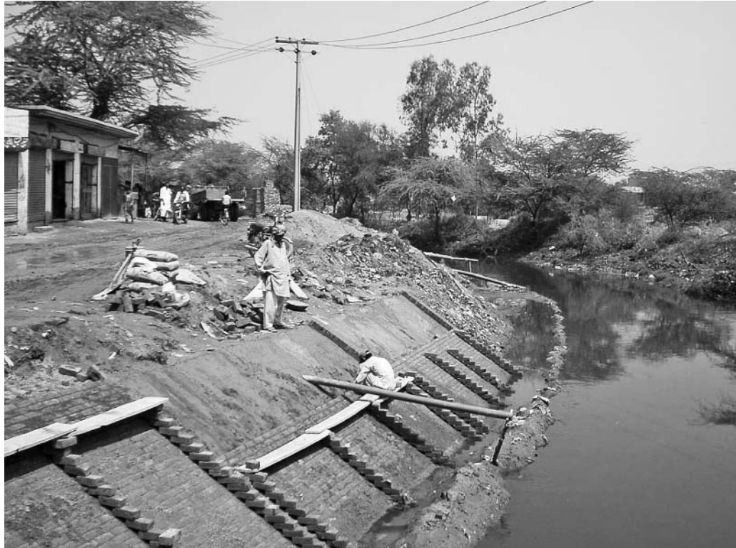
Photo 6.3: The retrofitting of a lining of local bricks along a drainage ditch in Lahore Pakistan. Accumulated debris, sediment and vegetation has been removed from the ditch, the bank re-profiled. Source: Peter Lingwood.
