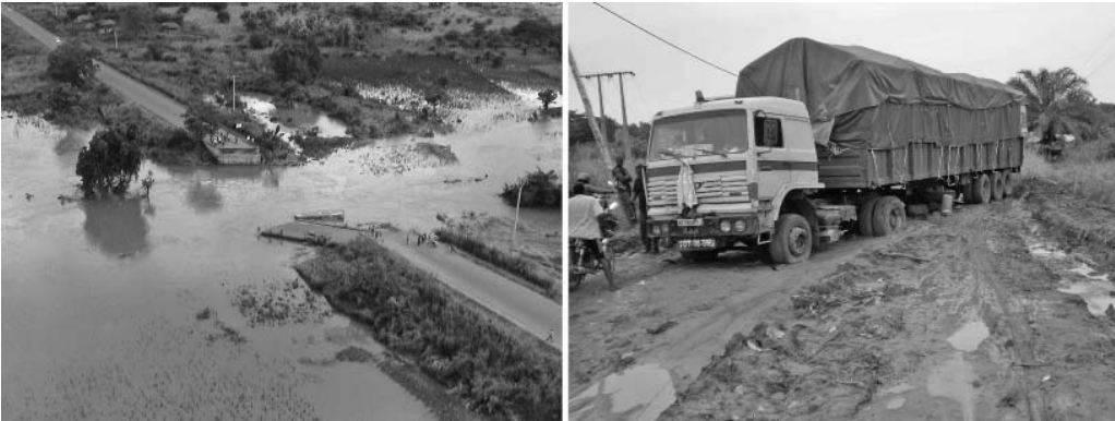
Photos 2.2 and 2.3: Roads destroyed in Togo, 2008. Source: Ayeva 2011
