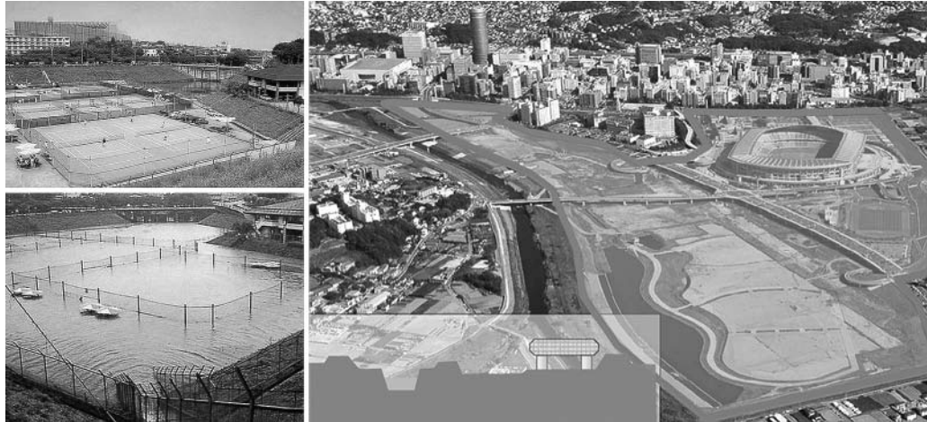
Figure 3.7: An outflow control facility and Tsurumi multi-purpose retaining basin. Source: Ministry of Land, Infrastructure and Transport, Japan; Tanaka 2011.
