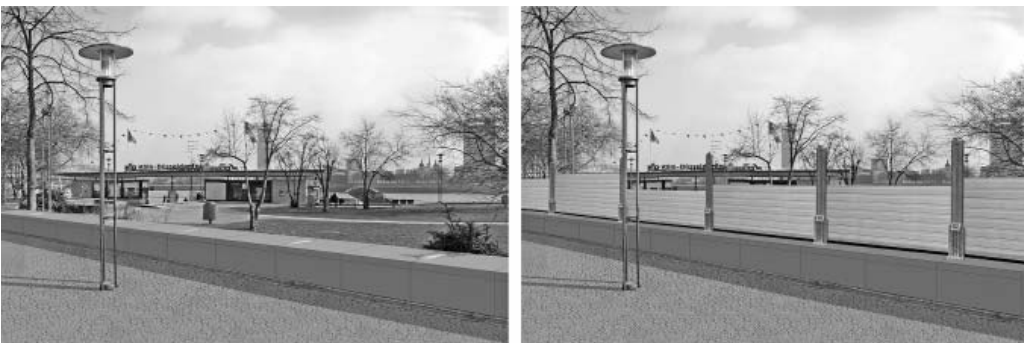
Figure 7.3: Raising and enhancing the existing flood protection with mobile walls. Source: Heinz Brandenburg, StEB
