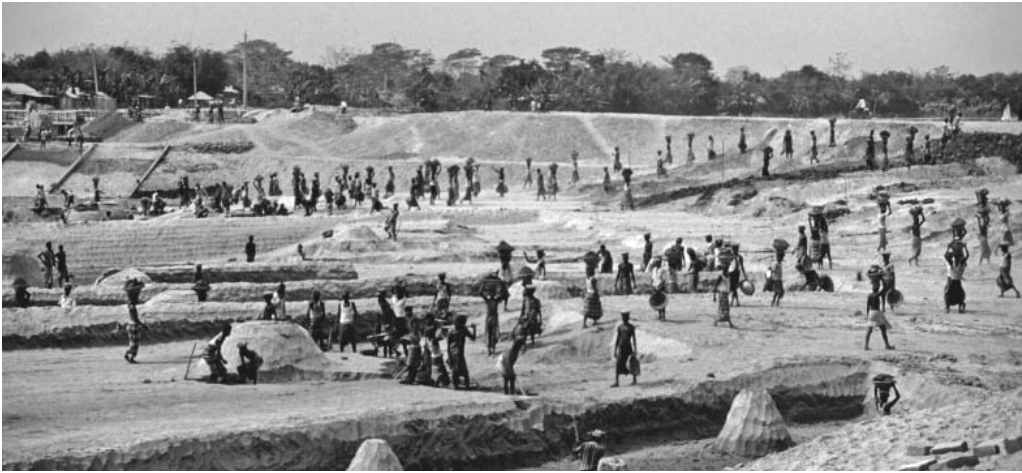
Photo 3.4: Labor intensive construction of river flood protection embankments in Bangladesh. Source: Alan Bird
