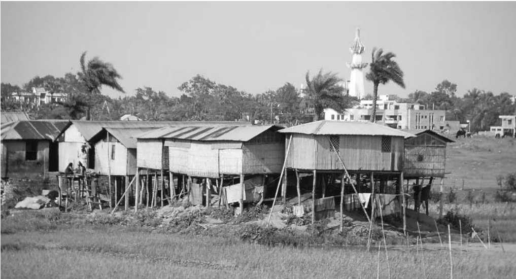
Photo 3.13: Houses raised on stilts to avoid flooding in Bangladesh. Source: Alan Bird.
